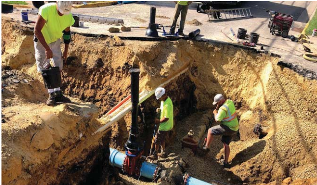
DODGEVILLE, WI, SPRING STREET RECONSTRUCTION
