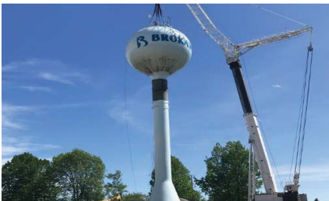
MAINE, WI, WATER SYSTEM IMPROVEMENTS
